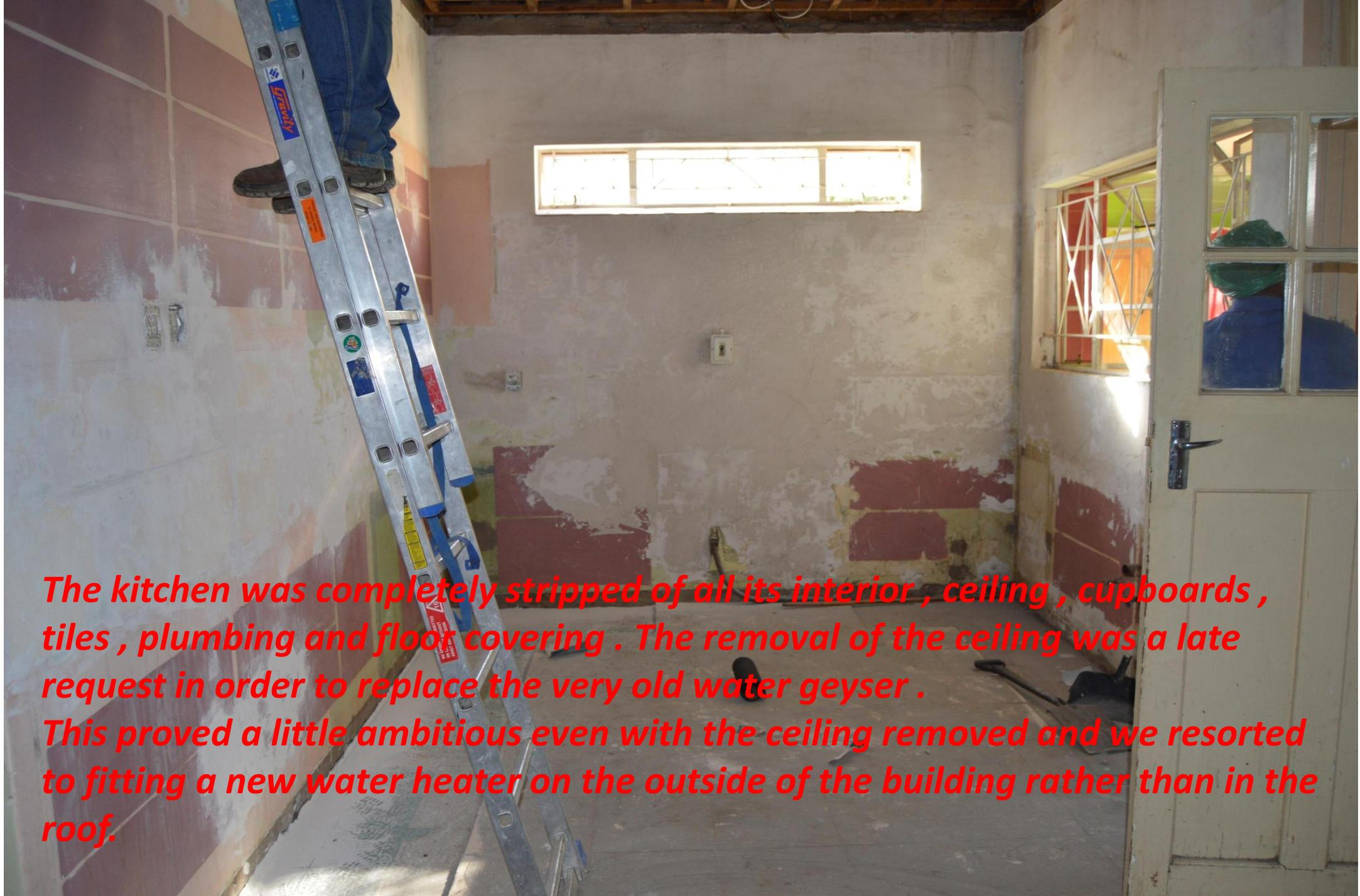
*The kitchen was completely stripped of all its interior , ceiling , cupboards , tiles , plumbing and floor covering . The removal of the ceiling was a late request in order to replace the very old water geyser . This proved a little ambitious even with the ceiling removed and we resorted to fitting a new water heater on the outside of the building rather than in the roof.*
